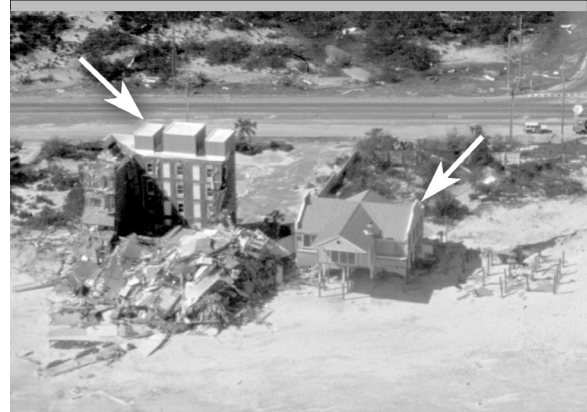
After the hurricane: The front of the 5-story building collapsed and the pilings under the house were exposed.
